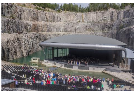
Figure 8: The new roof at Dalhalla. Photo: Per Frankelius.
